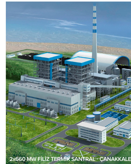
2x660 MW FİLİZ TERMİK SANTRAL - ÇANAKKALE
